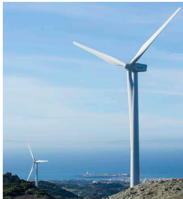
Repowering project El Cabrito, Tarifa, Spain. Completed in 2018. It was 25 years old when dismantled and resulted with 87% fewer turbines with the same output capacity. Source: ACCIONA.
