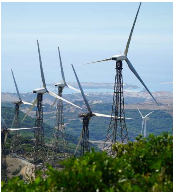
Repowering project El Cabrito, Tarifa, Spain. Completed in 2018. It was 25 years old when dismantled and resulted with 87% fewer turbines with the same output capacity. Source: ACCIONA.
