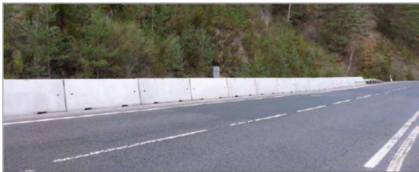
Precast concrete New Jersey barriers
